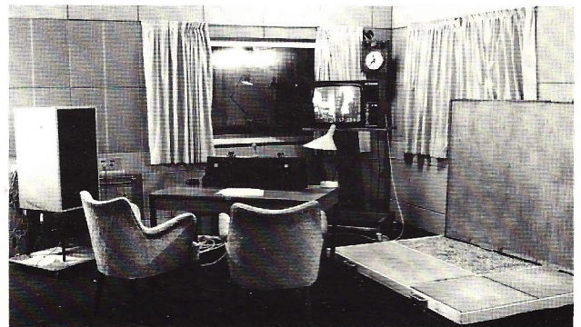
Fig. 10 Studio adjacent to Sypher suite, showing commentators' sound and picture facilities. On right, sound effects tray for footstep effects on gravel, stone, wood and linoleum.
