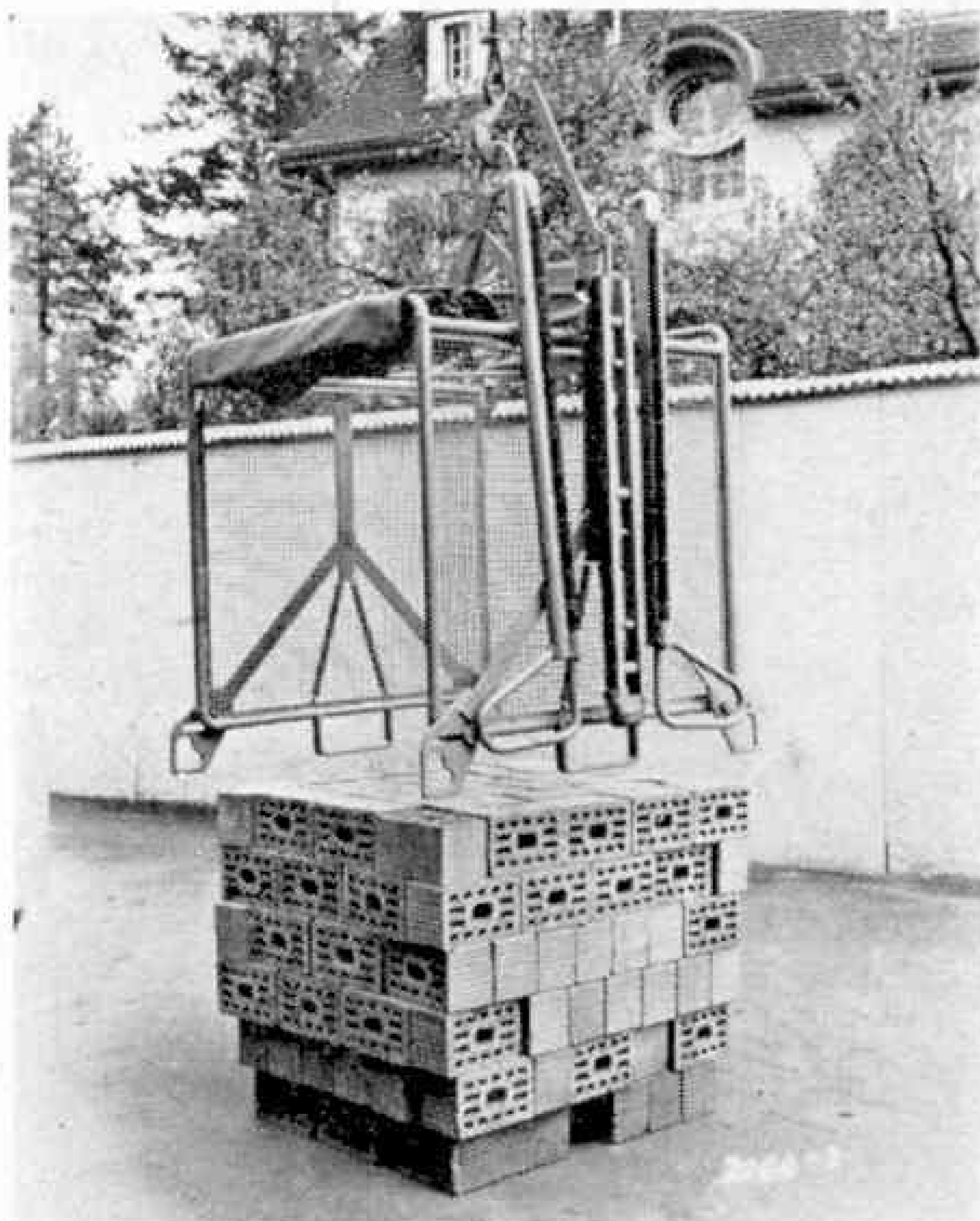
The crane grab about to close over a unit load of bricks. The photographs and the details on which this article is based are by courtesy of the Editor of Claycraft.
