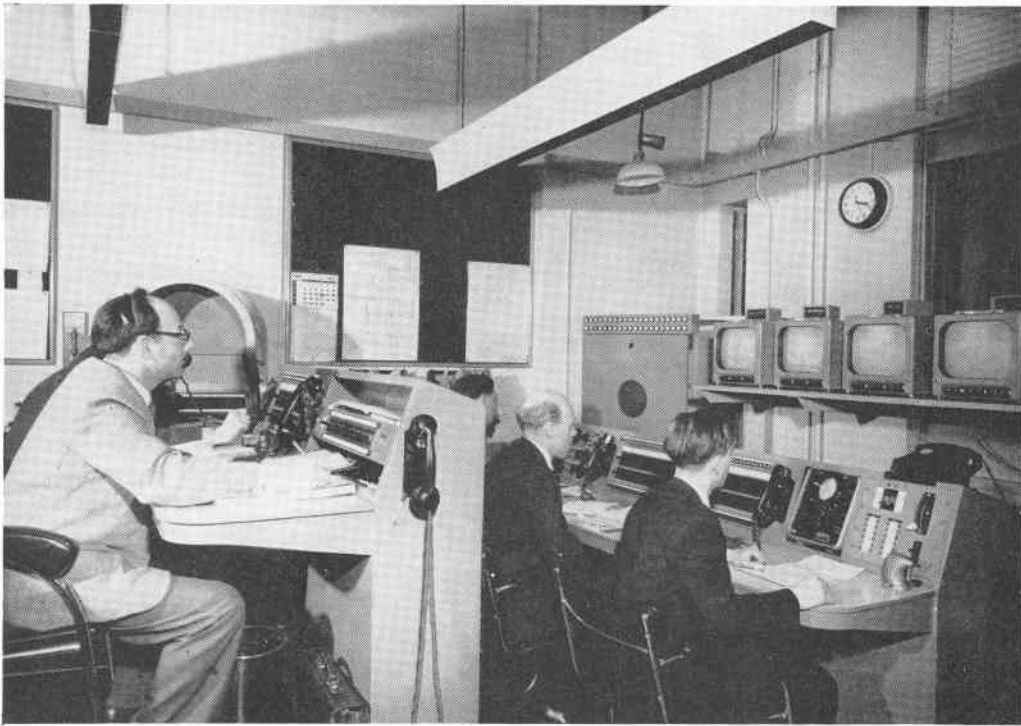
The Continental Control Point in Broadcasting House, London, through which pass the vision and sound signals of Eurovision programmes to and from the United Kingdom.
